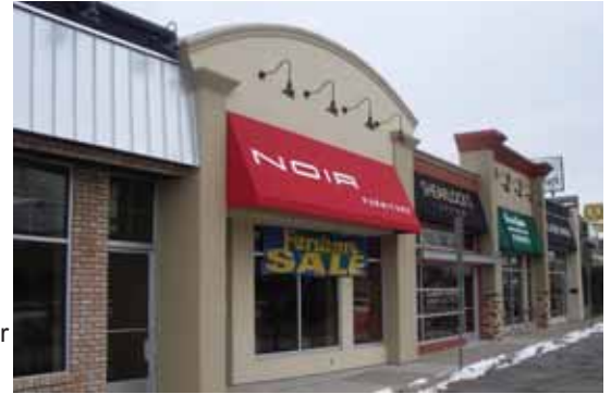
The new facades include lighting, large windows, and materials unique to each storefront.
